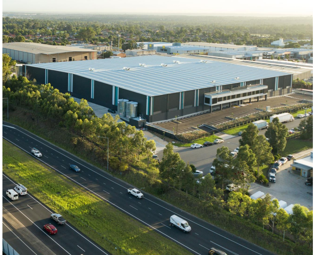
42 Cox Place, Glendenning, NSW.
